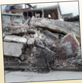
Unimaginable destruction caused by earthquake.
